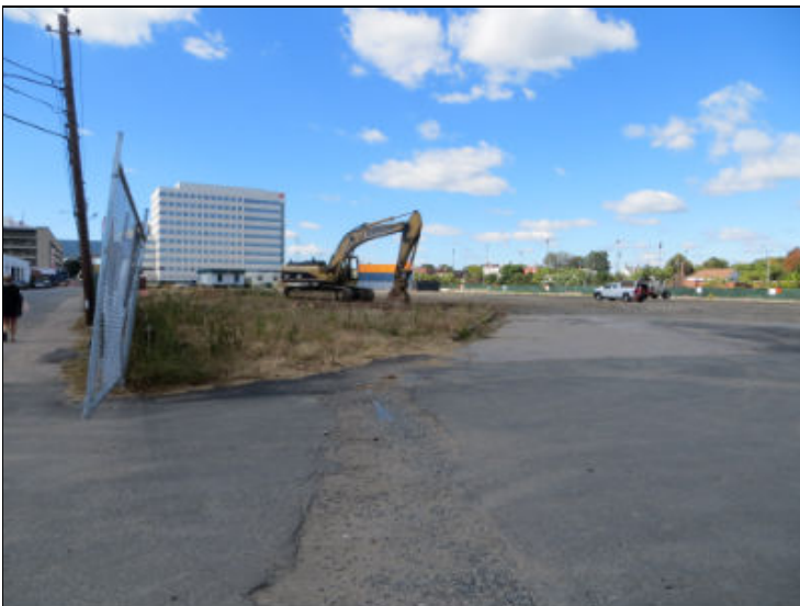
On Guest Street. New Balance is mobilizing for its $500M project.
